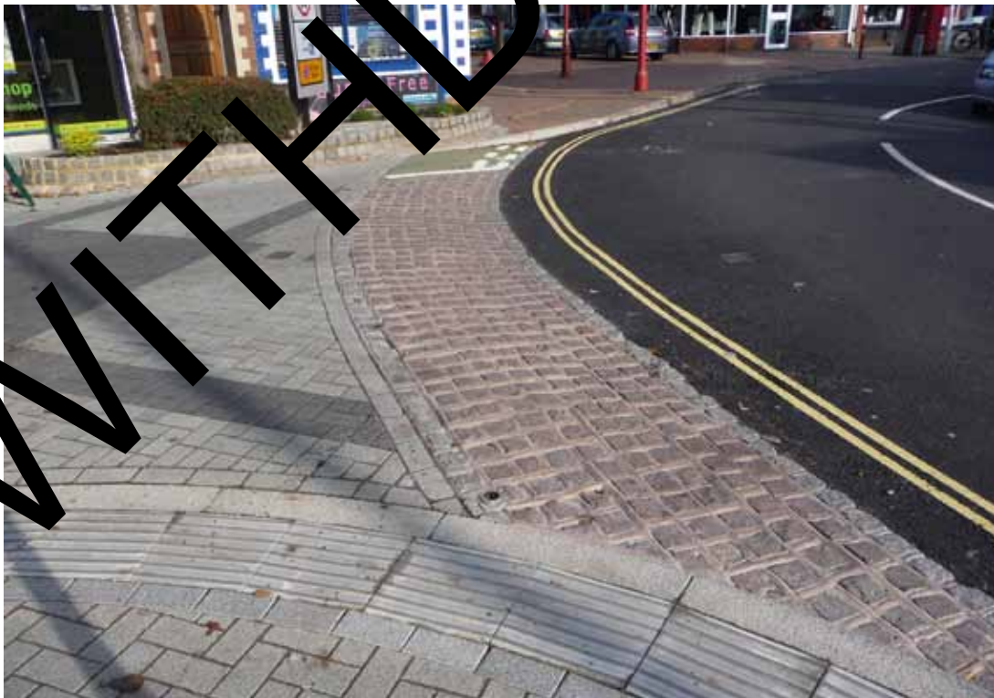
Figure 6.2 Example of a shared space gateway feature
