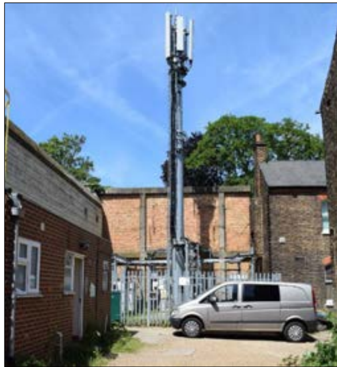
Photo 7: Telephone mast in south-west corner of site, view from east
