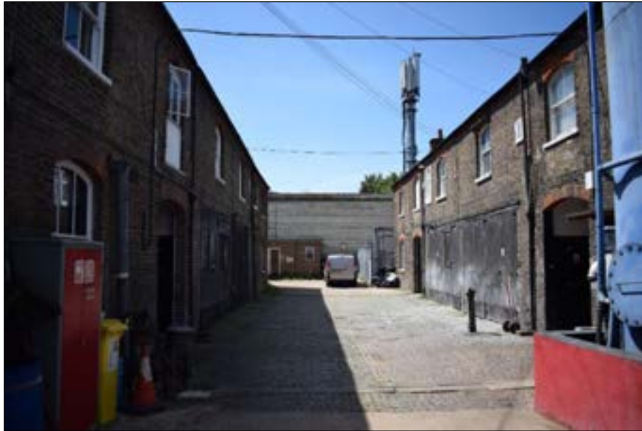
Photo 4: Victorian buildings and cobbled surface, view from north-east
