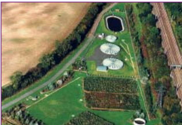
Sundon landfill leachate treatment plant, commissioned in summer 1997
