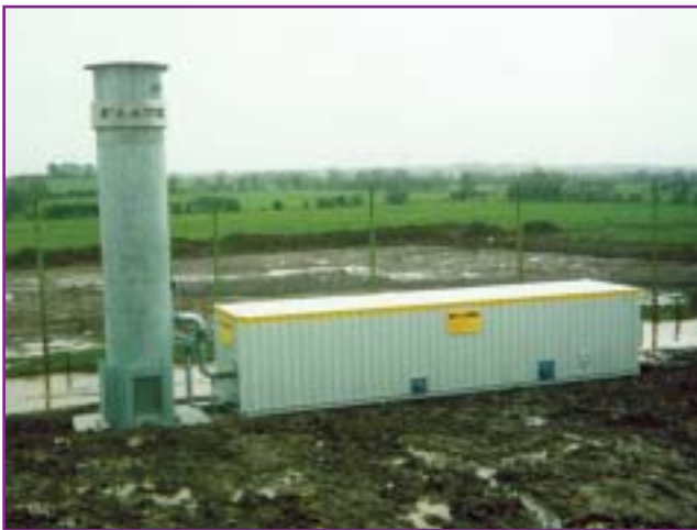
Basketstown Landfill Gas Plant, Co. Meath
