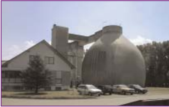
Anaerobic digestion plant in Germany
