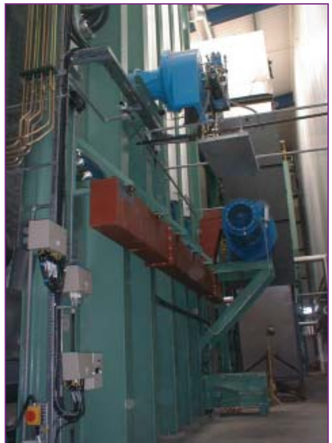
Boiler unit in small scale thermal treatment plant
