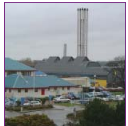
Bournemouth clinical waste incinerator
