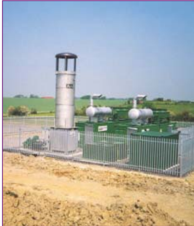
Typical small landfill gas compound
