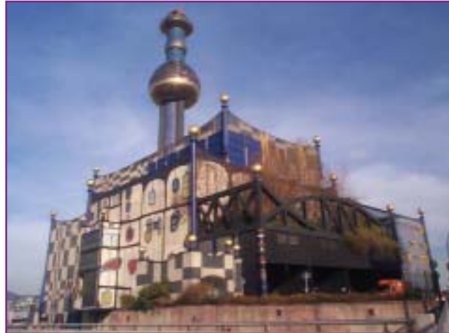
Vienna combined heat and power plant
