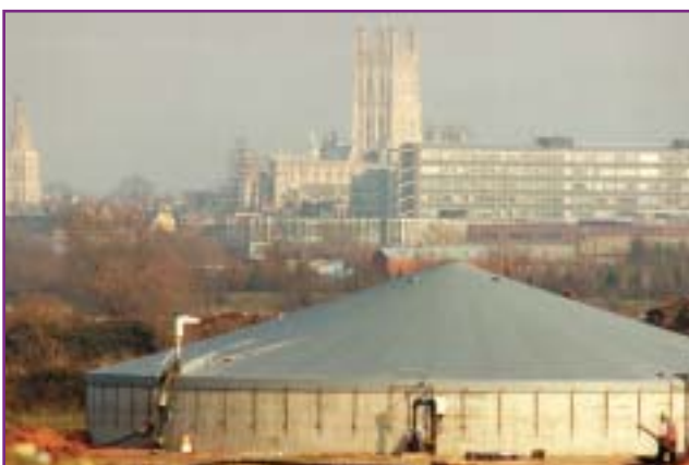
Hempsted landfill leachate treatment plant
