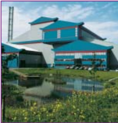
View of Billingham plant showing pond feature in foreground and architectural embellishment on main plant building
