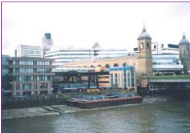
Wallbrook Wharf transfer station, central London
