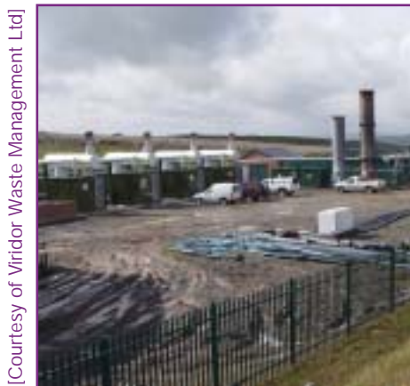
Pilsworth Power Plant
