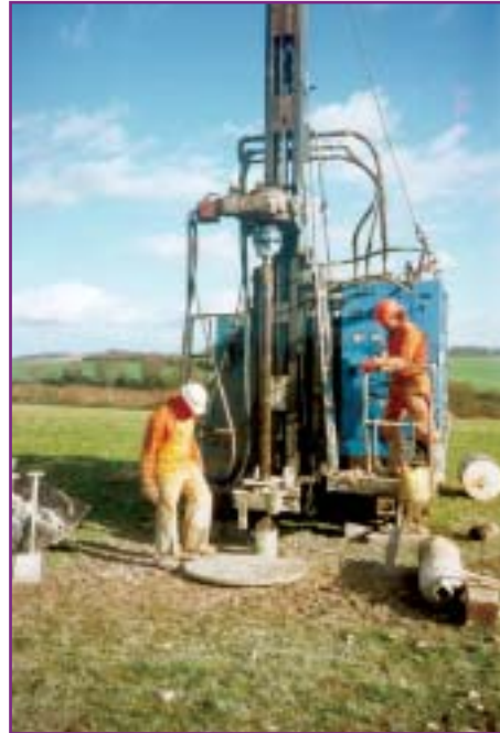
Installing a gas well
