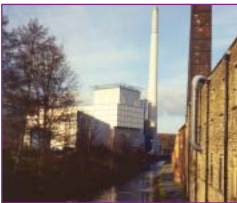
Actual view of Kirklees Waste to Energy plant
