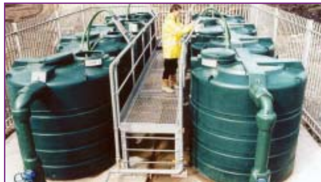
The configuration of a methane stripping plant at Red Moss Landfill Site, Manchester, where a series of individual 5000 litre aeration tanks are used in series to reduce the methane level by a factor of 100.
