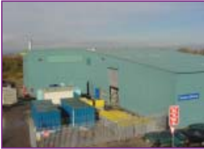
Compact Power facility, Avonmouth, Bristol
