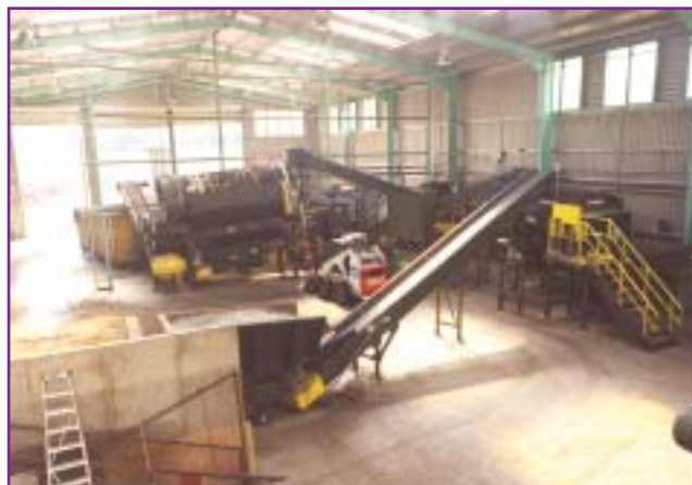
Mixed waste processing equipment
