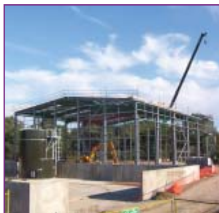
Wanlip AD plant under construction, September 2003
