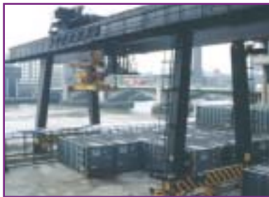
Walbrook Wharf Waste Transfer Station
