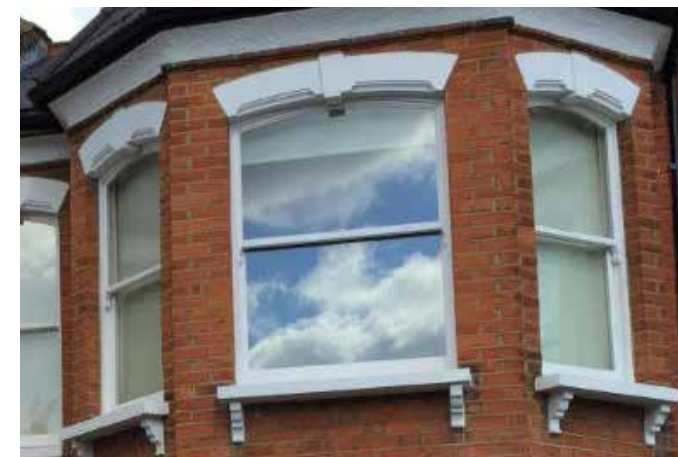
Timber sash window in a Victorian house
