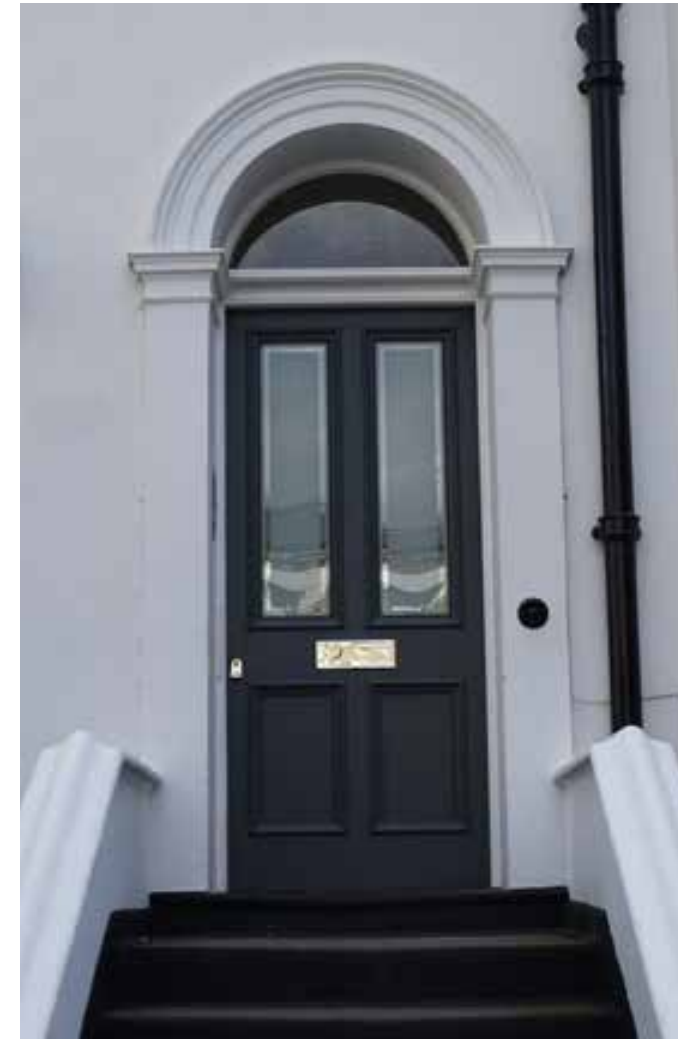
Timber panelled double doors with curve fanlight
