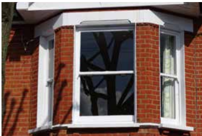
Timber sash window in a c. 1900 house
