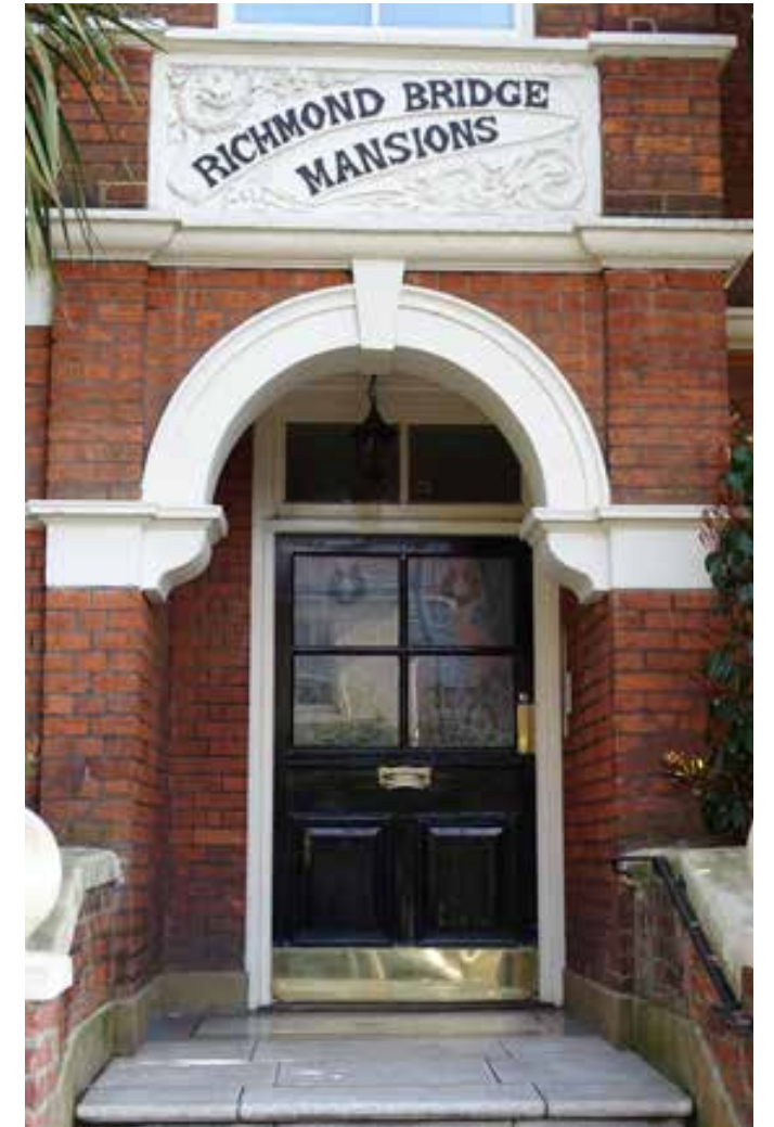
Timber panelled door in a c. 1900 mansion block
