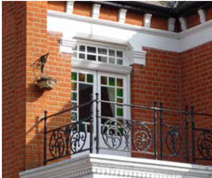
Timber casement balcony doors with Iron railing balustrade
