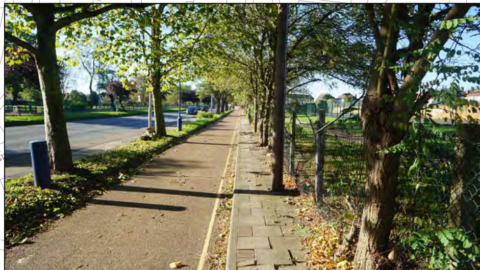
Existing service road to be raised level with the footway and both footway and service road to be surfaced in a buff coloured material. This will provide a 4m wide shared surface.
