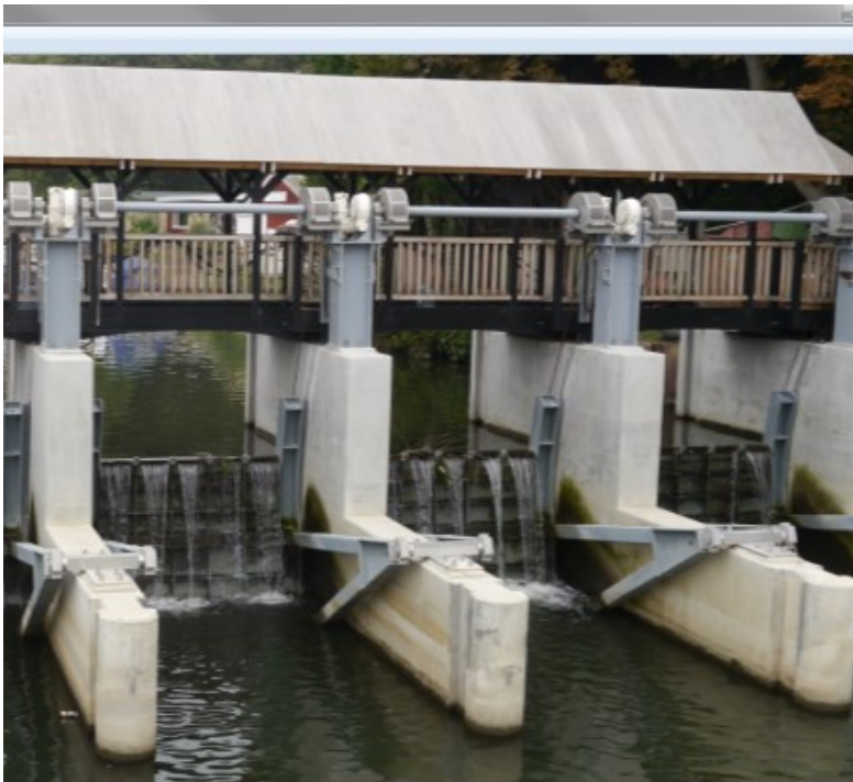
Figure 4-8: Example of a fixed weir radial gate.
