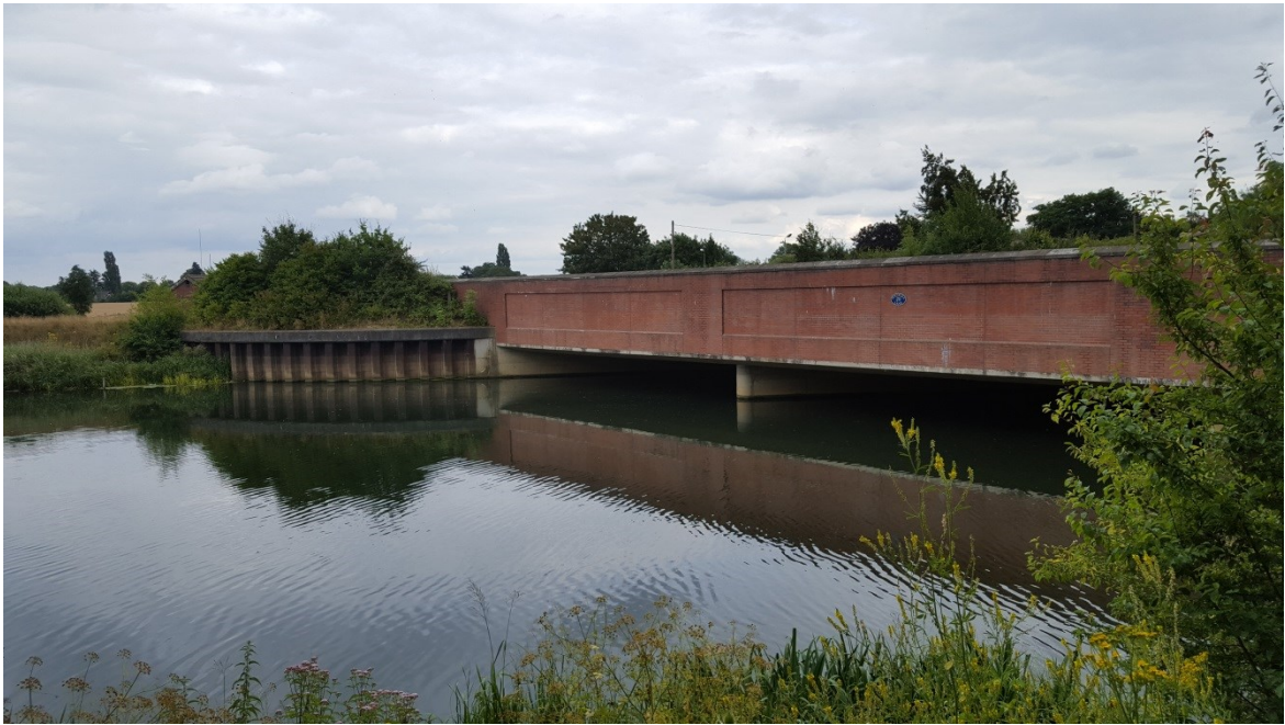
Figure 4-4: An example of a typical culvert.
