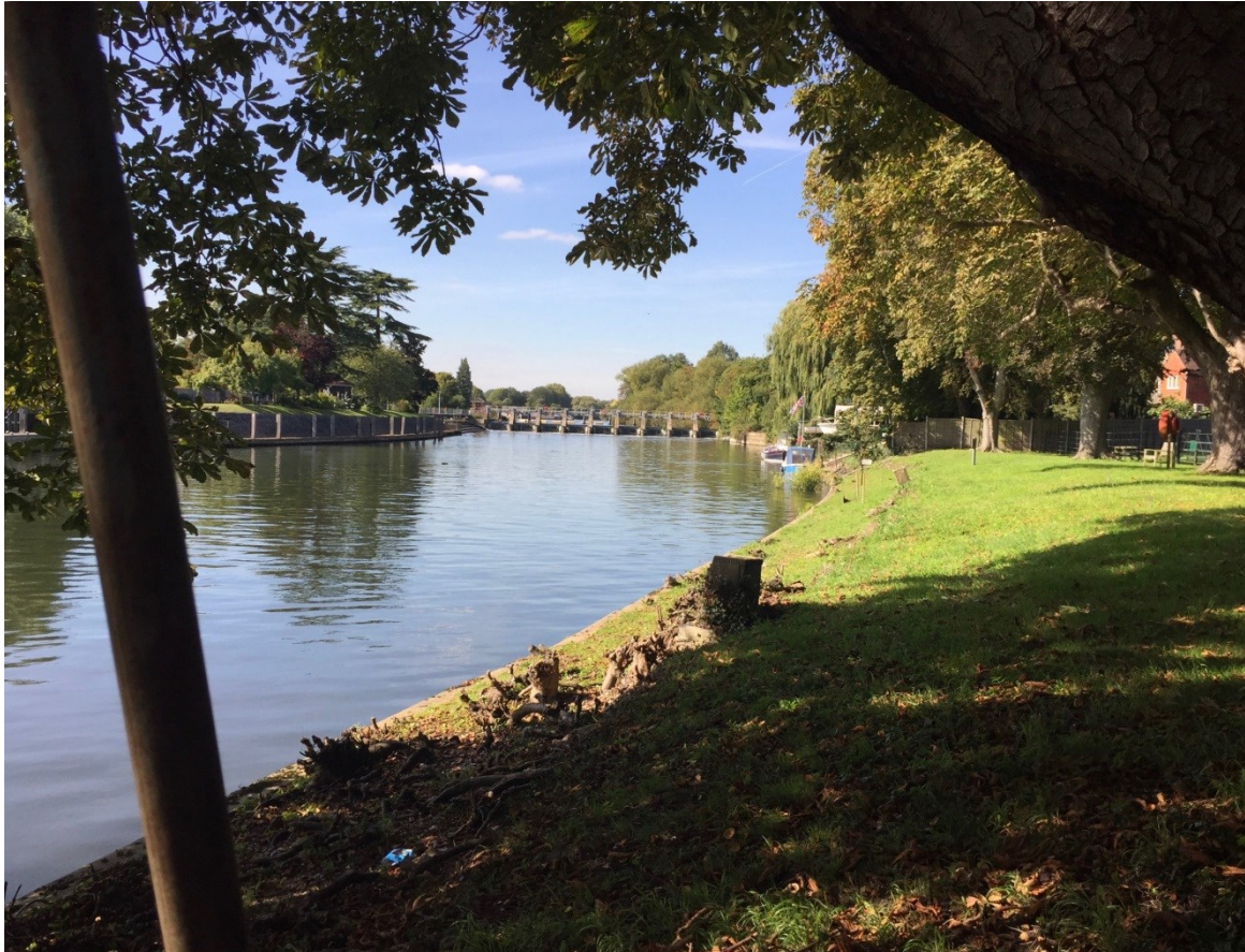
View of Bell weir on the River Thames at Hythe End, from downstream of the Channel Section 1 outlet.
