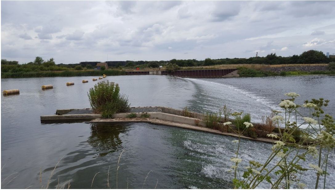
Figure 4-6: An example of a typical water level control structure.
