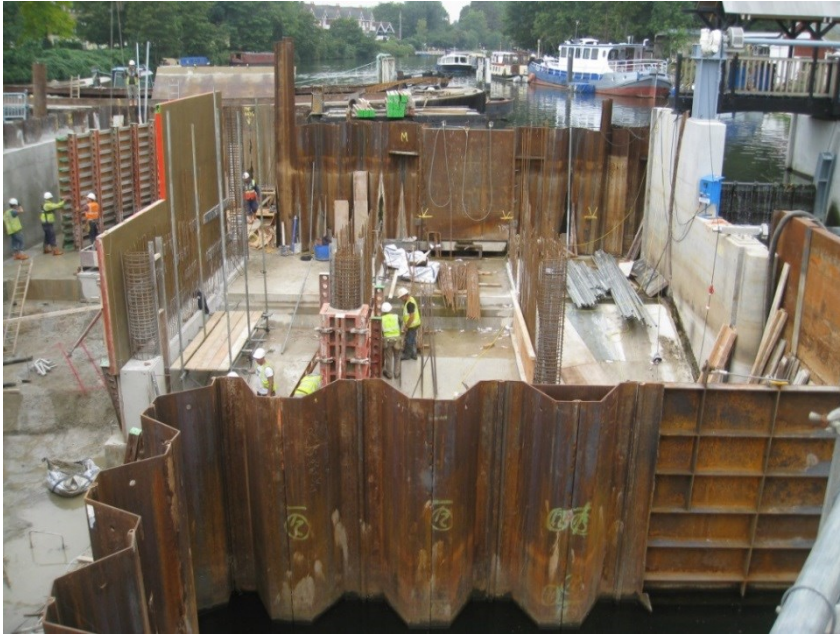
Figure 4-10: An example of a cofferdam, used to construct new weir gates.
