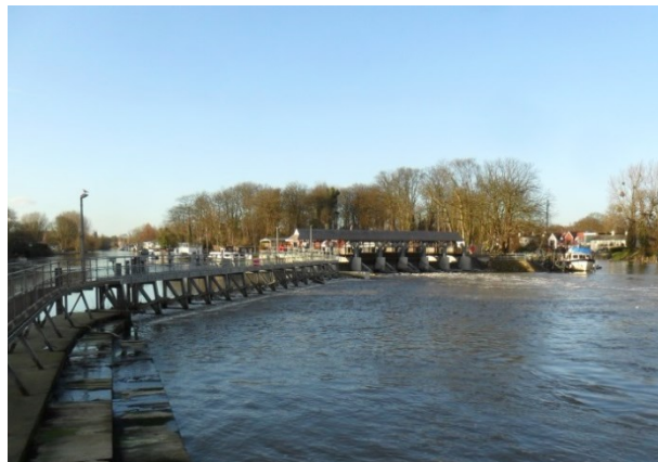
Figure 0-4: Molesey weir - where new gates will be built with a canopy similar to the existing.
