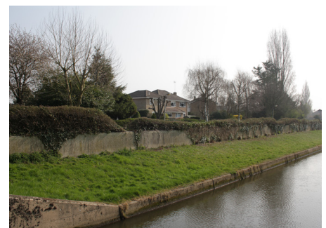
Properties overlooking Thames Water abstraction channel
