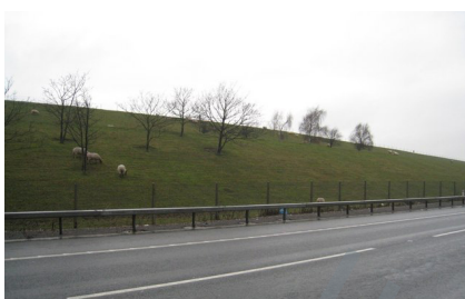
Sheep grazing on the embankment
