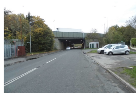
Wraysbury Road crossing under the M25
