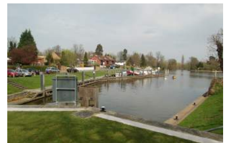
View from Shepperton Lock House
