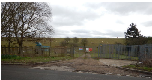
Wraysbury Reservoir Service Entrance
