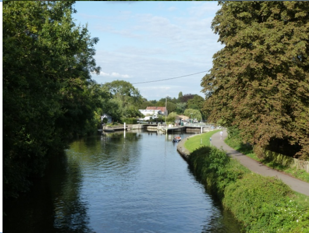
Photograph 10: Sunbury lock, looking east. Horse chestnut tree potentially suitable for roosting bats on south bank of the Thames. Vegetation growing on soft banks of the Thames
